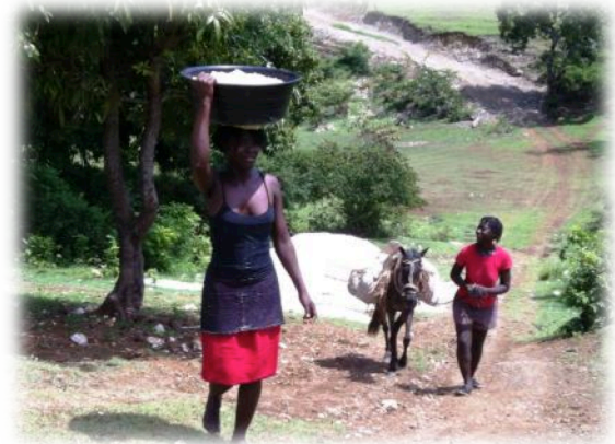
After digging the foundation, the families carry materials on their heads, using a donkey and a horse.
